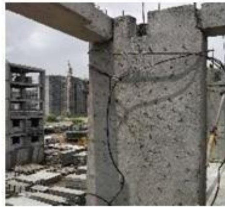
Figure 16. Notch connection
