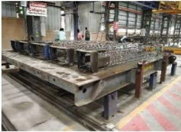
Figure 5. Reinforcement with notch plate
