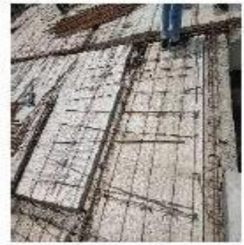
Figure 19. slab to slab connection
