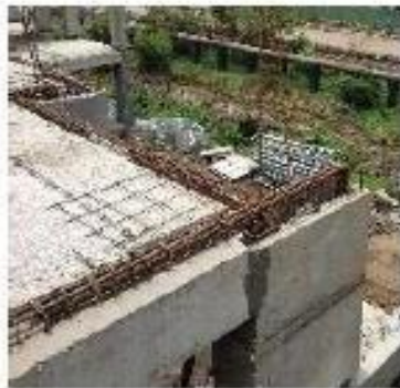
Figure 17. Column to beam connection
