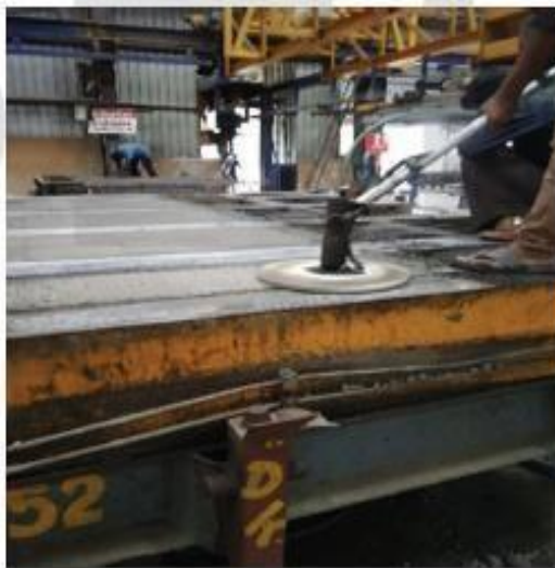
Figure 7. Finishing with floater machine
