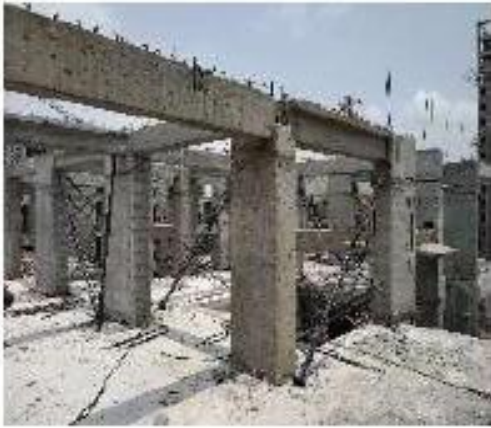
Figure 15. Beam resting over column
