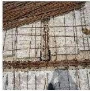
Figure 18. Beam to beam connection
