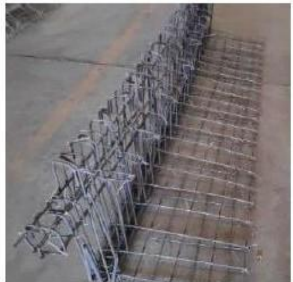
Figure 2. Beam Reinforcement
