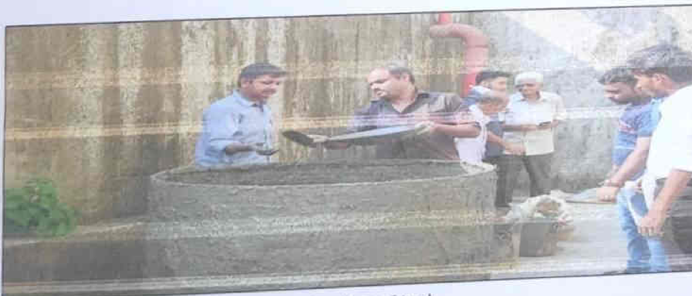
Construction of tank
