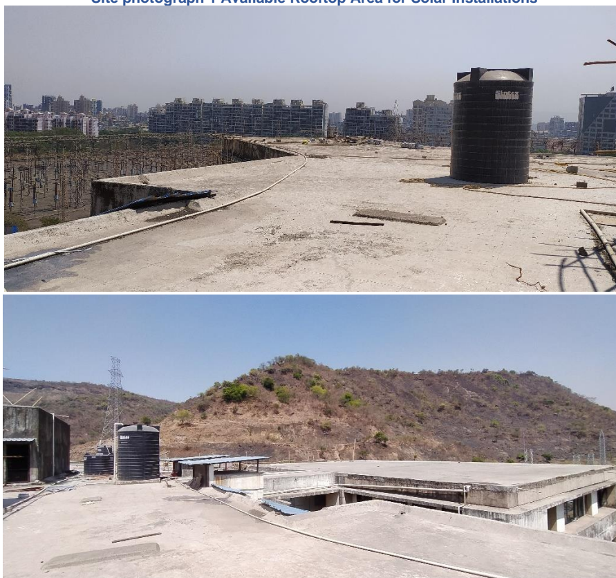
Site photograph 1 Available Rooftop Area for Solar Installations
