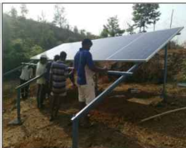
Installation of 2 set of solar panel for the purpose of pumping water to the villagers through solar energy
