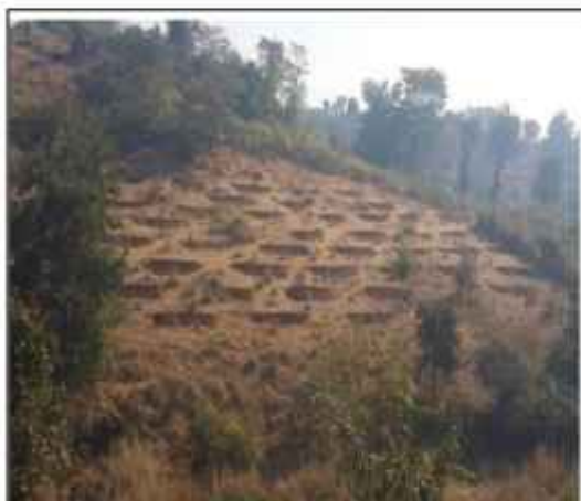
75 CCT (Continuous Contour Trenches) constructed to increase the water level
